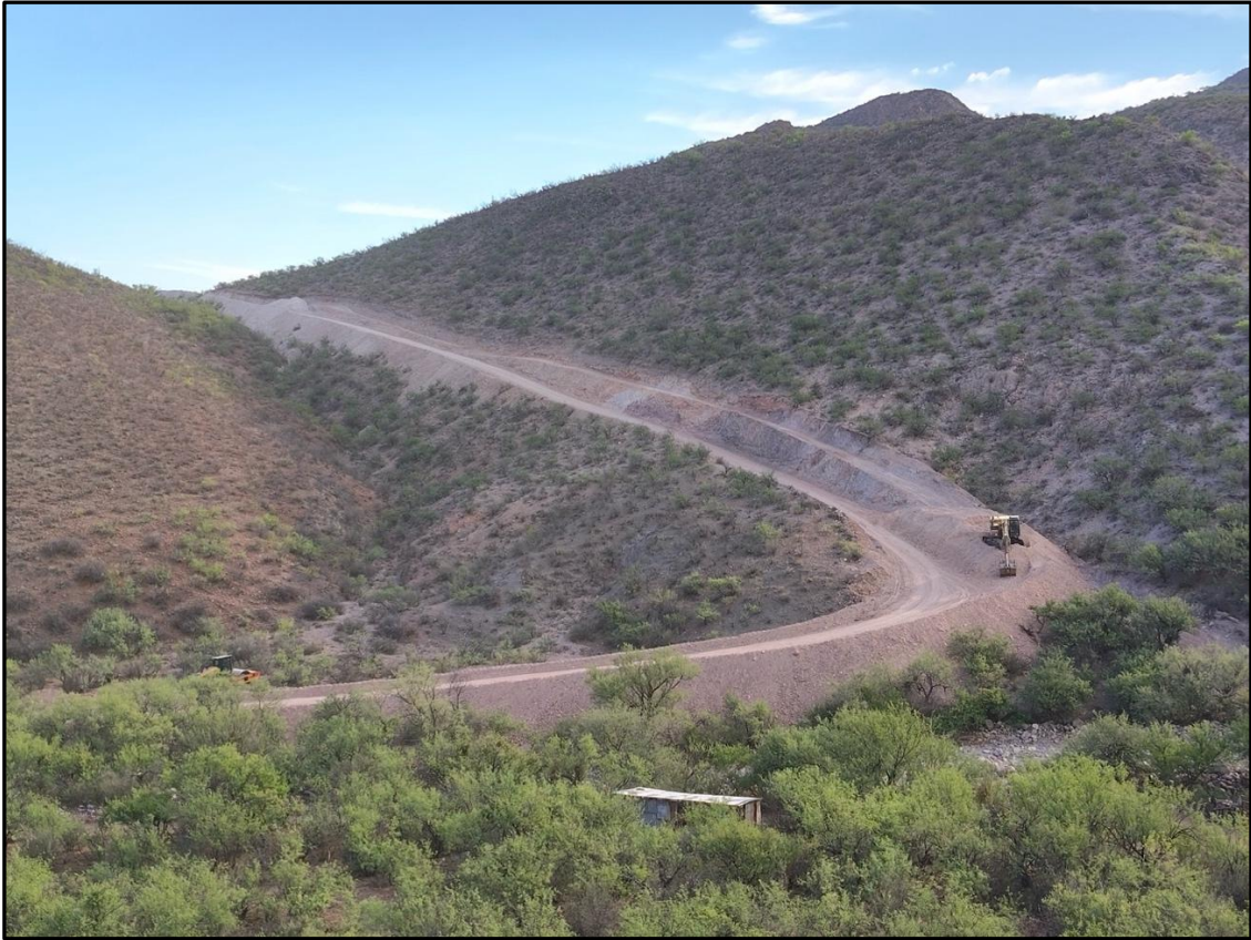
Photo 1: Rehabilitation of Main Access Road for Full Freight Haulage
