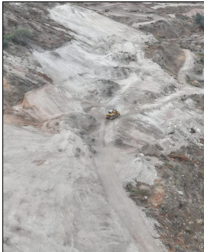
Photo 4: Earthworks at the Merrill-Crowe Plant and Pregnant Pond Areas
