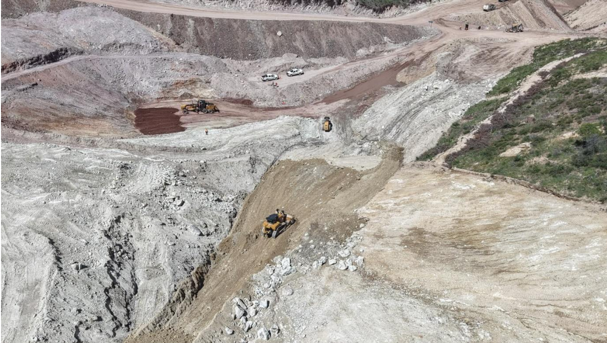
Photo 3: Earthworks of the mine facilities are 30% complete.
