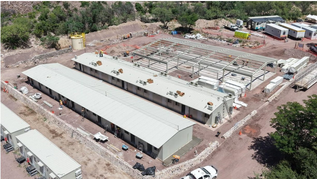
Photo 2: Construction of the mine operations camp is 50% complete.
