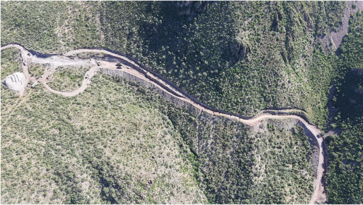
Photo 1: Improvements to main access road are 85% complete.
